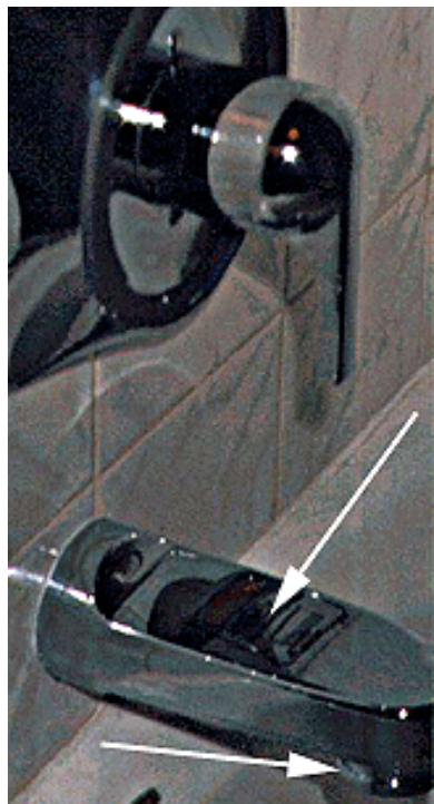
Figure 2.14: Hidden shower control. To divert water to the shower, you have to pull down on the knob beneath the faucet. [Photograph courtesy of Baddesigns.Com [Darnell 2010].]
