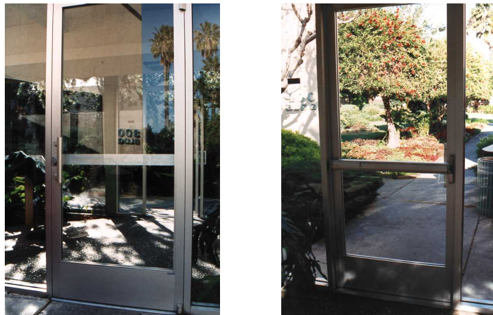
Figure 2.20: Good use of affordances in the same hotel. This door is well designed. The vertical handle correctly suggests pulling, the flat bar correctly suggests pushing.
